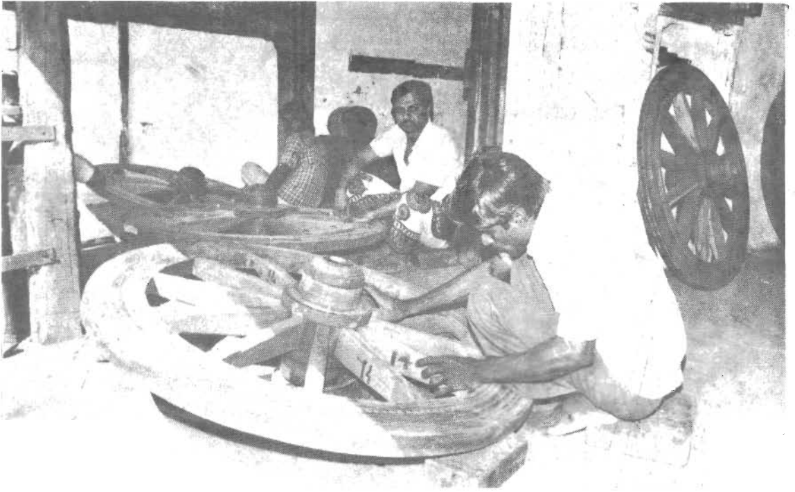
Plate No. 38 Bullock Cart Wheel Manufacturing
