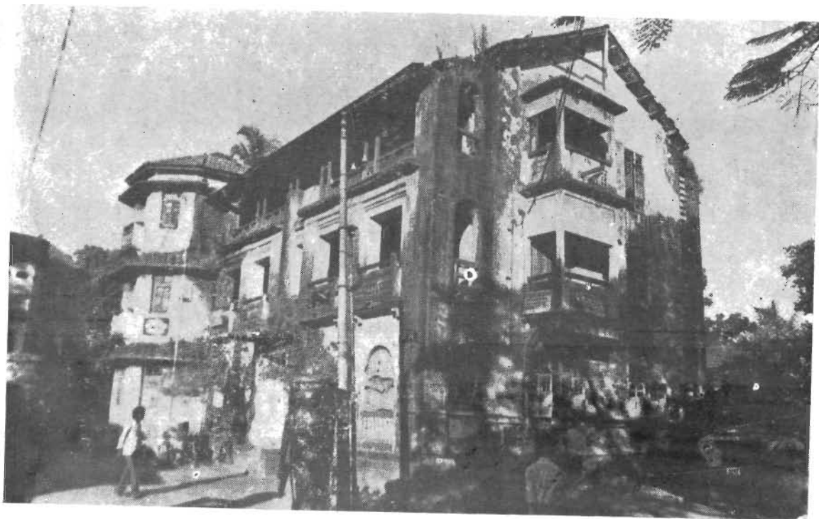
Plate No. 8 Panchayat Samiti Office
