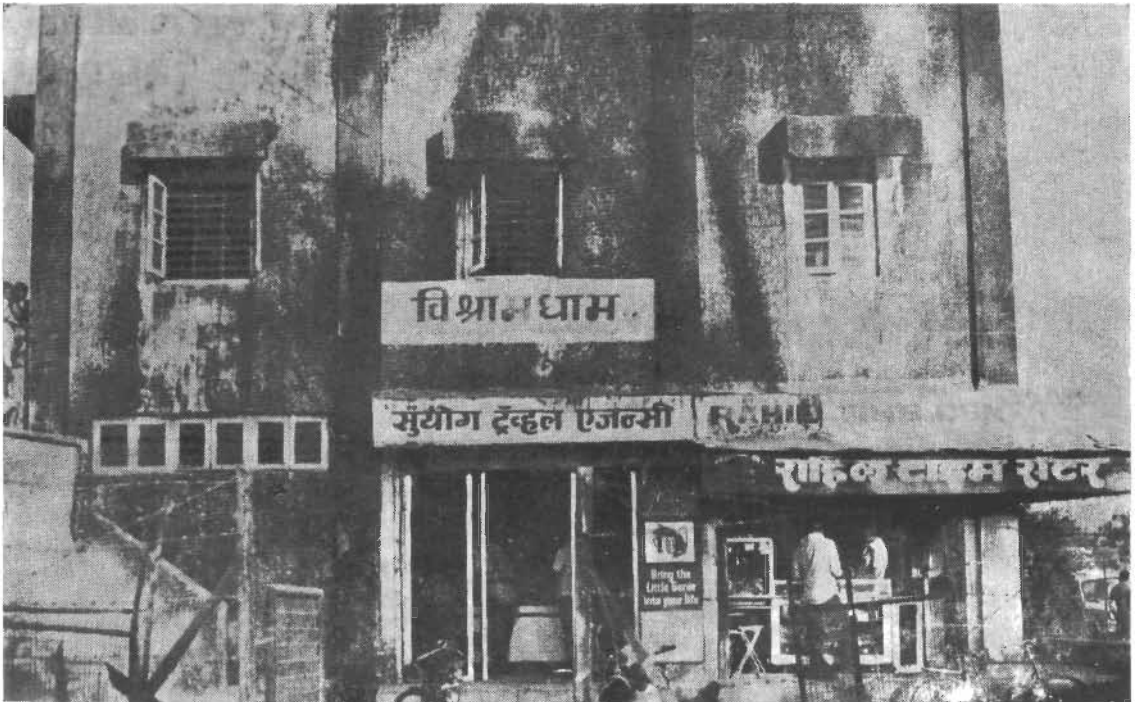
Plate No. 20 Revenue Rest House
